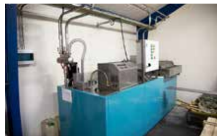
The central filtration system for filtering coolant.
